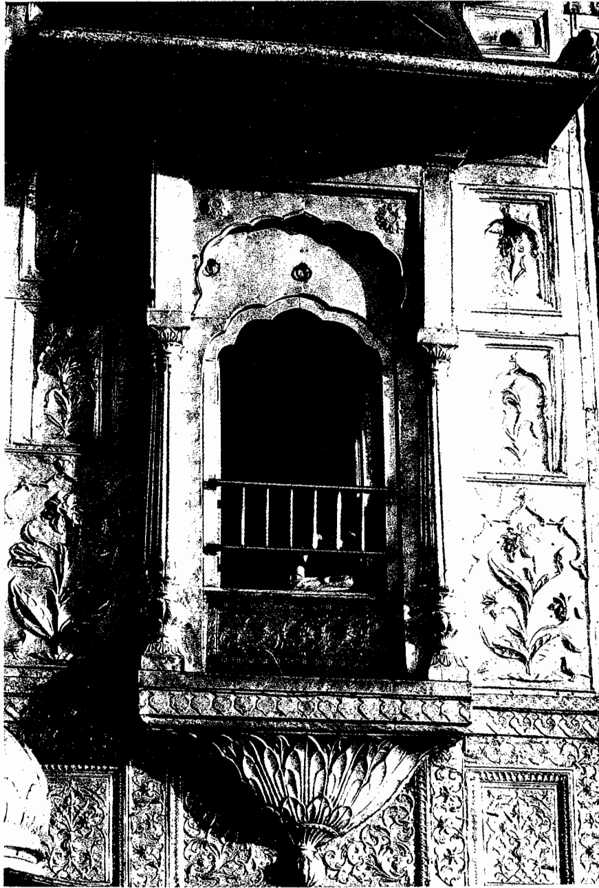
Platé 13. An óriel window from the western facade.
